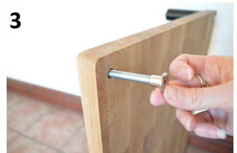
Fit the stud assembly through the wood panel
